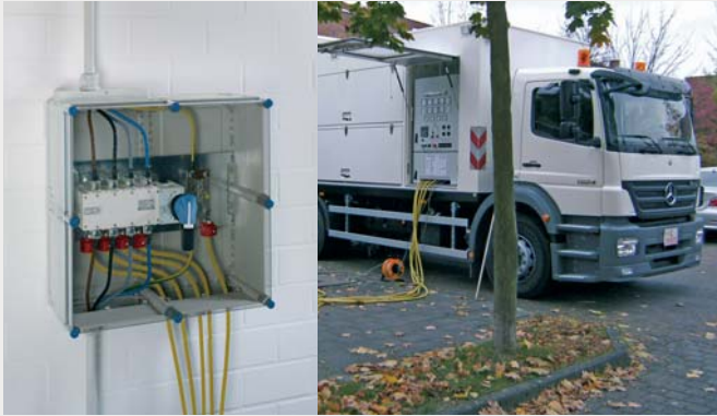
Changeover switch boxes (I-0-II) switch safely to substitute power sources
